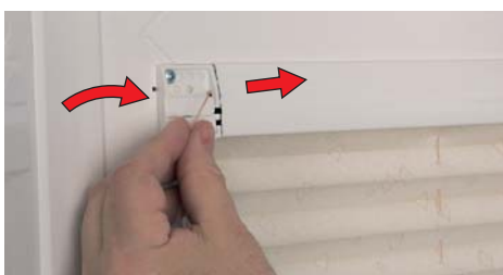
13. Press locking gate closed to secure cord. Cut-off excess cord leaving 100mm min. Tuck through hole in endcap
