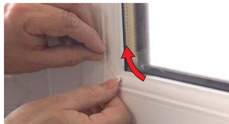
11. Holding button, pull cord tight to secure
