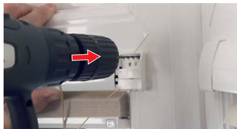
8. Drill Ø2.5mm holes 2 off on each side
