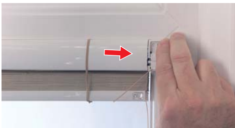
7. Stick blind onto frame leaving rubber band around blind
