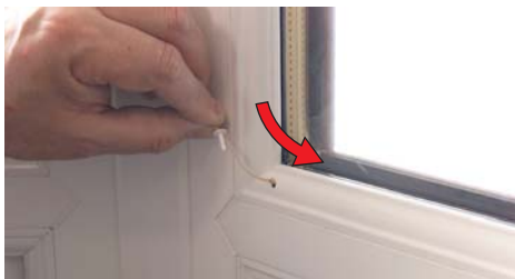
10. Push cord knot into hole, push fixing grommet into hole, aligning groove to cord
